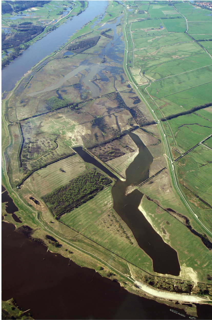
FIGURE 8 | Aerial view of the Middle Elbe River Levee Setback and River Restoration Project in the Lenzen Area (Germany) (courtesy of Katharina Nabel).
